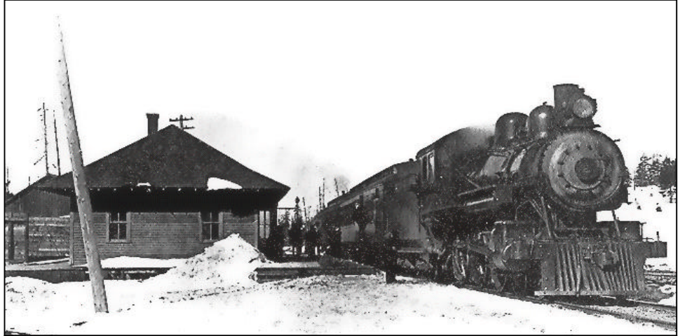
Alco 4-6-0 No. 2 rests at the Deary depot. With a construction number of 40685, she was the saturated-steam sister of the more popular super-heated No. 1 (c/n 40684). No. 2 was scrapped at Potlatch in the early 1950's.— HPG Collection
