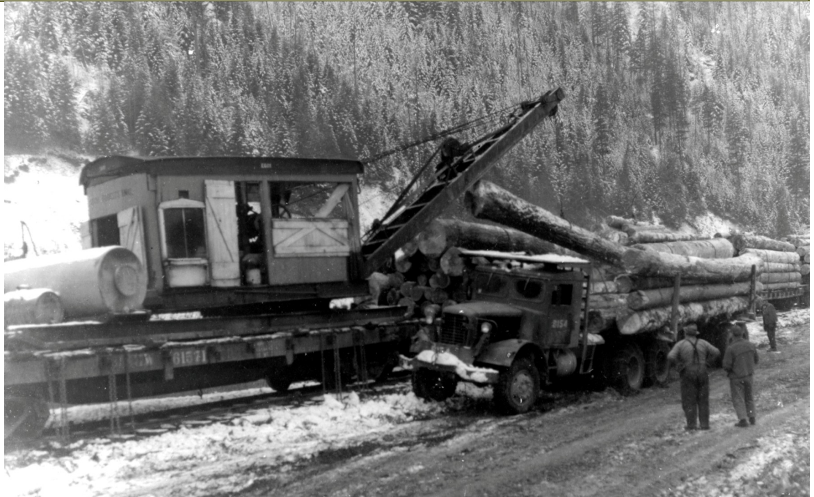
A PFI crew works to transload logs from truck to flatcar with a "slide-ass" diesel loader at this siding alongside the Milwaukee Road mainline a mile west of Avery. The St. Joe River flows between the tracks and the hillside in the background.
