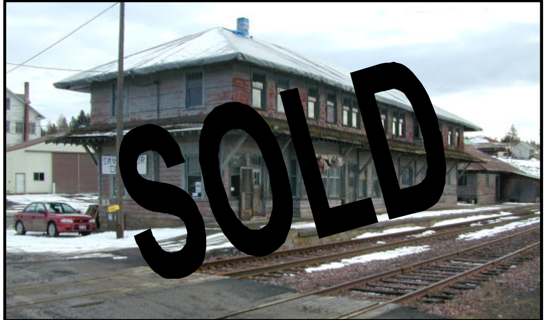
The Potlatch Depot is awaiting its restoration and renovation into an integral part of Potlatch daily life. This February 10 digital photo was included in the $500,000 Depot Enhancement application delivered to the Idaho Transportation Dept. on February 16. HPG
