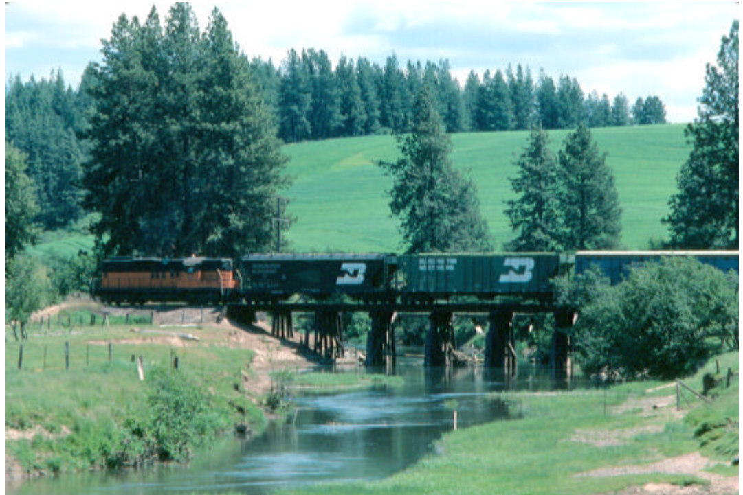
Eastbound WI&M freight behind Milwaukee Road GP-9 #280 (or 290) crosses bridge #2 just west of Kennedy Ford. This photo, taken in June 1976, shows the second incarnation of bridge #2, having originally been built as a Howe truss. The bridge was again rebuilt after this photo when several bents were damaged during the flooding of 1996. Carl Sonner photo
