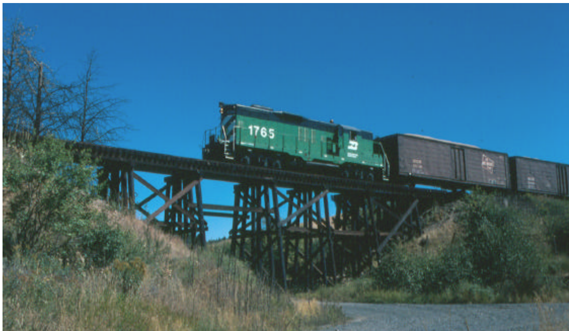
A Burlington Northern GP-9 hauls a trainload of Milwaukee Road rib-side boxcars converted into woodchip gondolas across WI&M bridge number 14 near Vassar, ID. Over the years, the WI&M replaced many of its trestles with fills, but having a road passing underneath probably saved this one from the same fate. Carl Sonner shot this photo in September, 1981.
